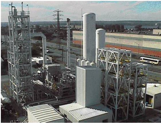
Figure 2.6. Atomic Energy of Canada Ltd. advanced heavy water pilot plant, Hamilton, ON. Photo courtesy Atomic Energy of Canada Ltd. This plant produced about 1 ton of heavy water per year. A scaled up version of it would be more efficient and cleaner than the old Bruce Point plant, shown above.
